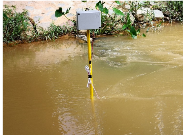
Figure 11: Prototype of Flood Detection with IoT is Located at River
