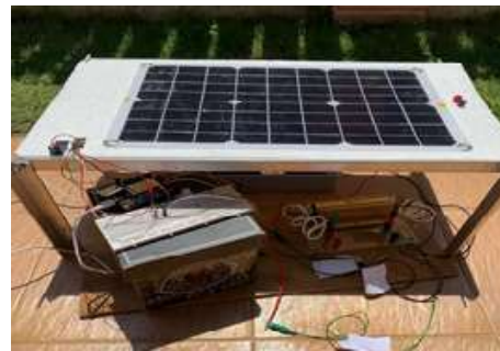
Figure 16: Prototype Stand-alone Wireless PV Monitoring System
